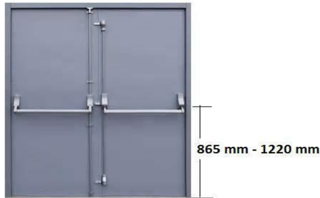
Figure 3.4.: Panic Hardware height from the finished floor
